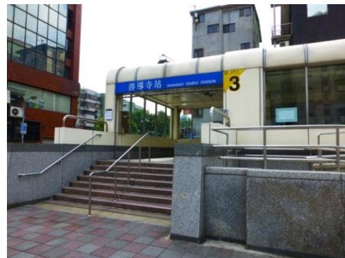
*MRT station in Taipei has a raised entrance against flood.
