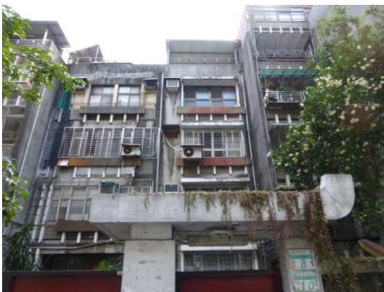
*Old apartment building constructed during the high economic growth period.
