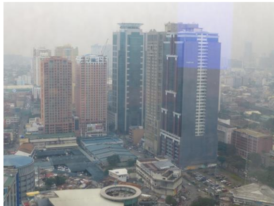
*Large scale condominium
