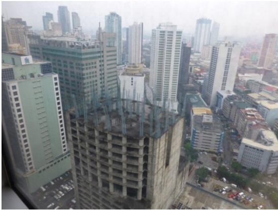
*A building which has halted construction
